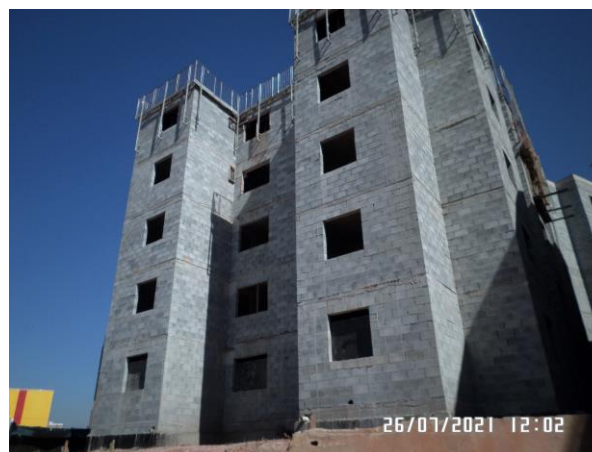
Vista Alvenaria - Cond. 6b
