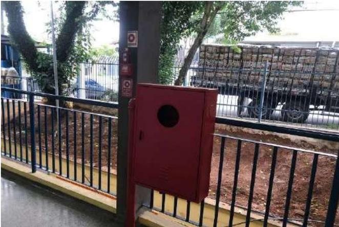
FOTO 157 HIDRANTE SEM COMPONENTES.
