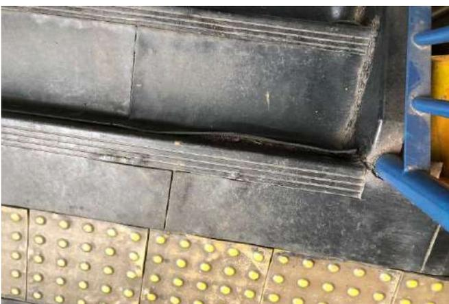
FOTO 131 ESCADA METÁLICA, COM PISO SOLTO.
