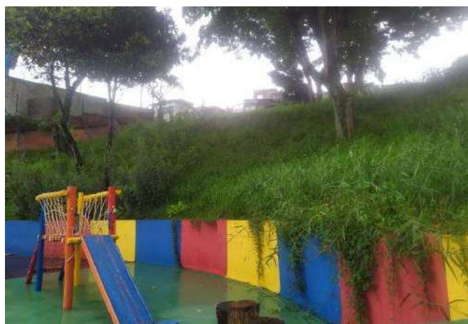
FOTO 46 Talude atrás do playground.
