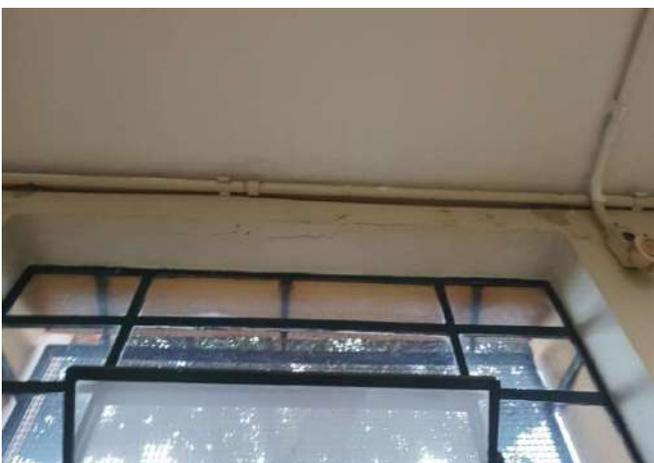
FOTO 59 CORREDOR INTERNO, FISSURA SOBRE CAIXILHO.
