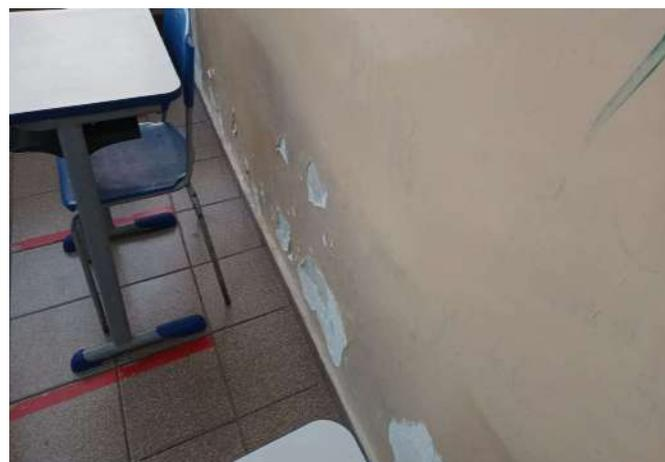
FOTO 82 SALA DE AULA 04 UMIDADE NA PARTE INFERIOR DA PAREDE
