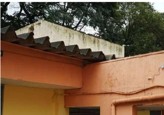
FOTO 119 ÁREA EXTERNA UMIDADE NA PLATIBANDA
