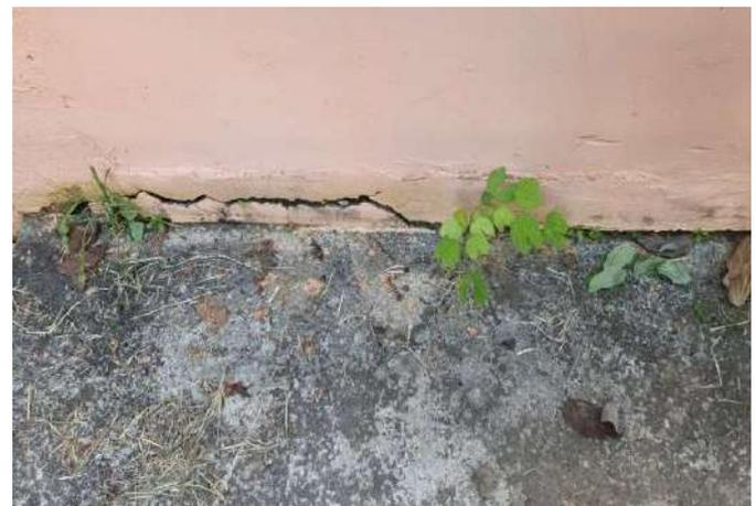
FOTO 22 PASSEIO INTERNO, PISO APRESENTA RECALQUE.
