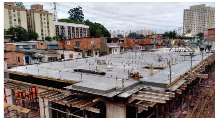
Vista do Cond. D – Bloco A e B
