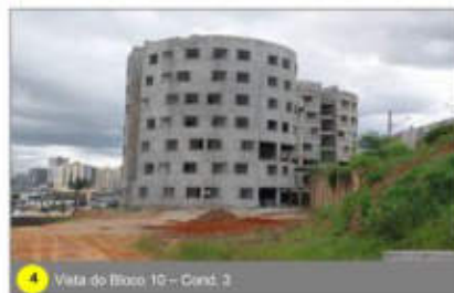
4 Vista do Bloco 10 – Cond. 3
