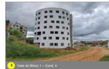
3 Vista do Bloco 1 – Cond. 4
