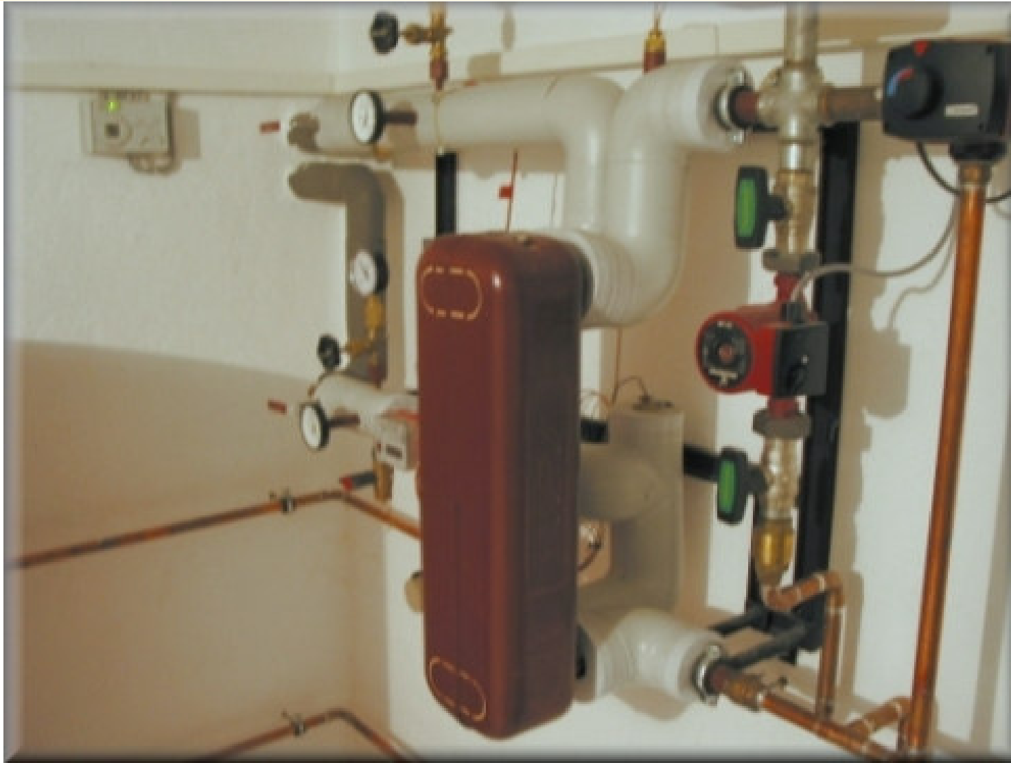
transfer station (basement)
