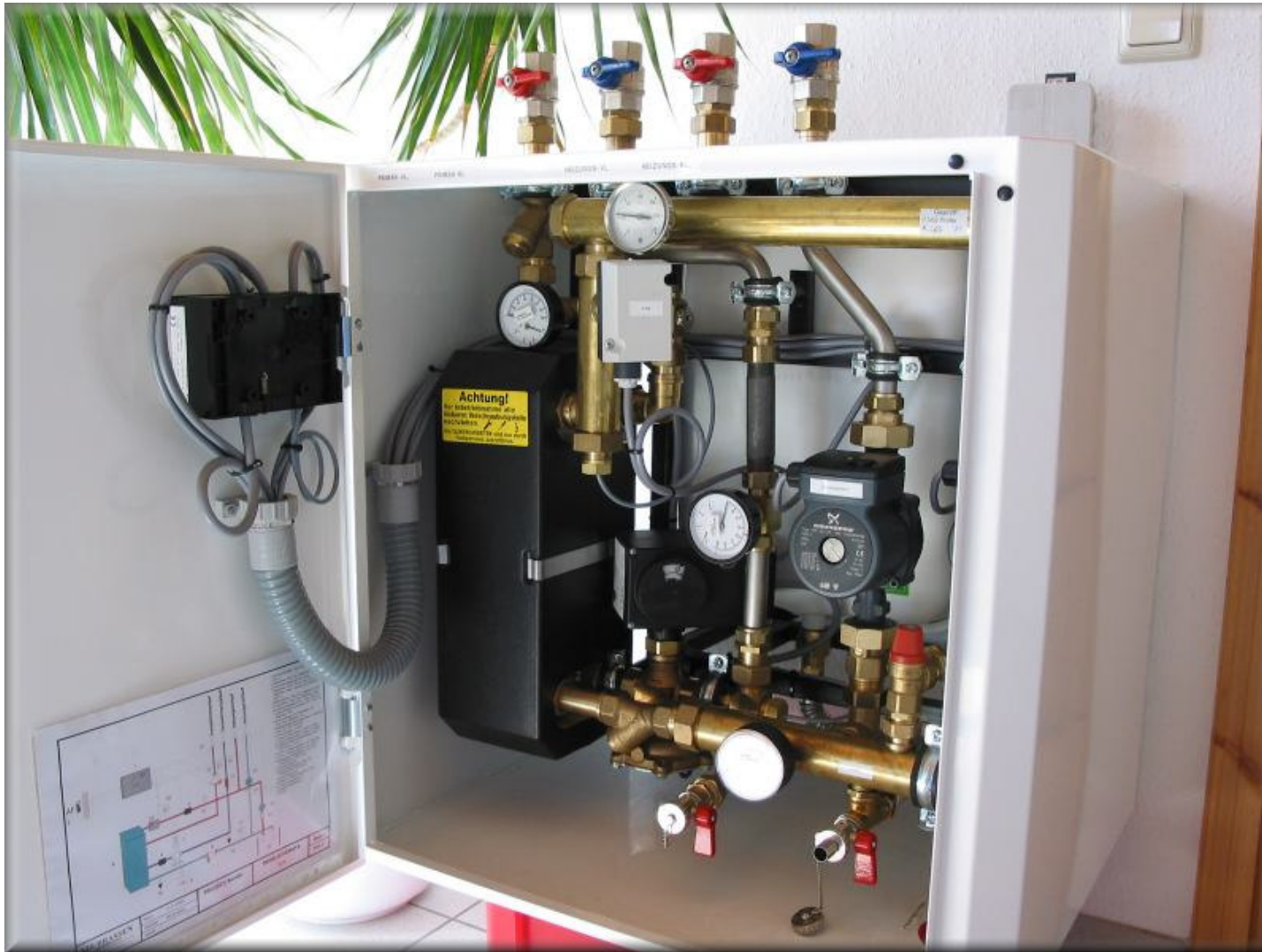
tight transfer station
